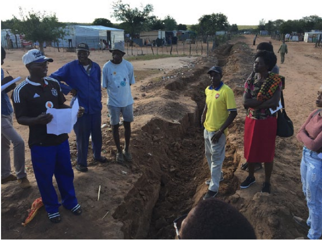
PHOTO 1 Digging of trenches for the infrastructure in Gobabis
